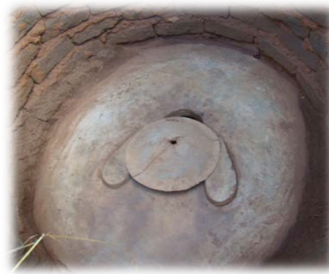
Figure 4-5: Domed slab with footrests and drophole cover in Msenda, Lilongwe district
